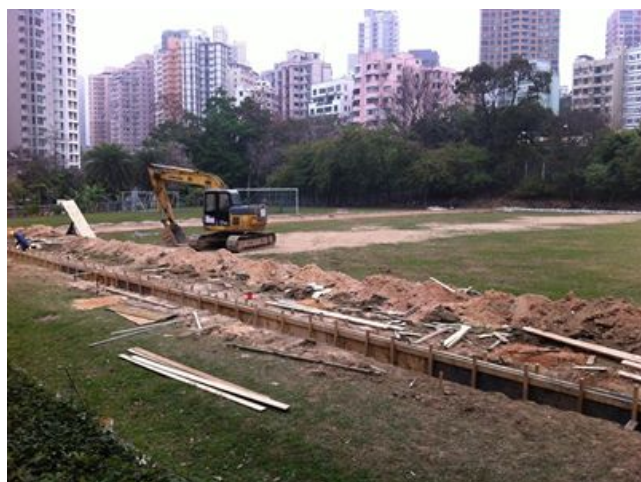
Works going on!
