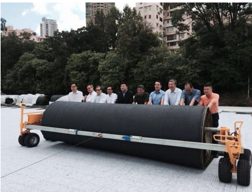
Laying the first roll of turf
